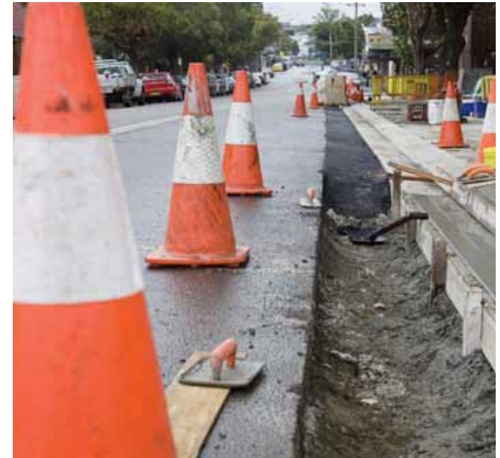
Repairing Parramatta's roads and footpaths is a never ending task.
