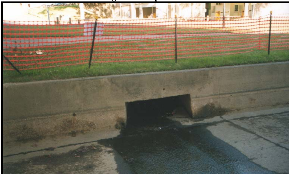
Photo 5 Box culvert draining the Phillip Lane and CBD catchment
